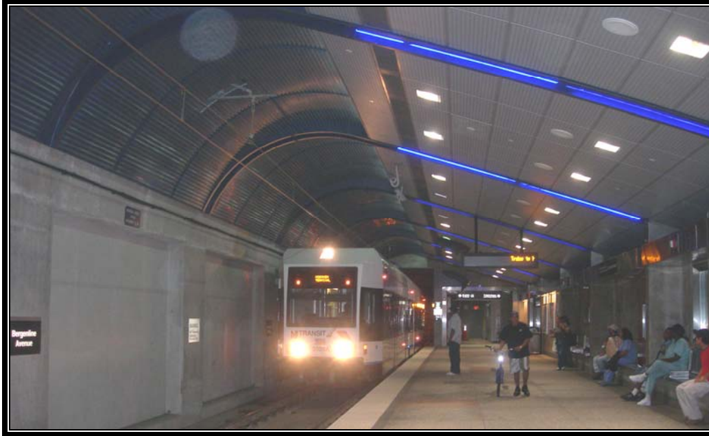
Bergenline Avenue Station platform level
