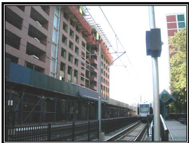
800 Jackson under construction at 9 th Street Station, Hoboken
