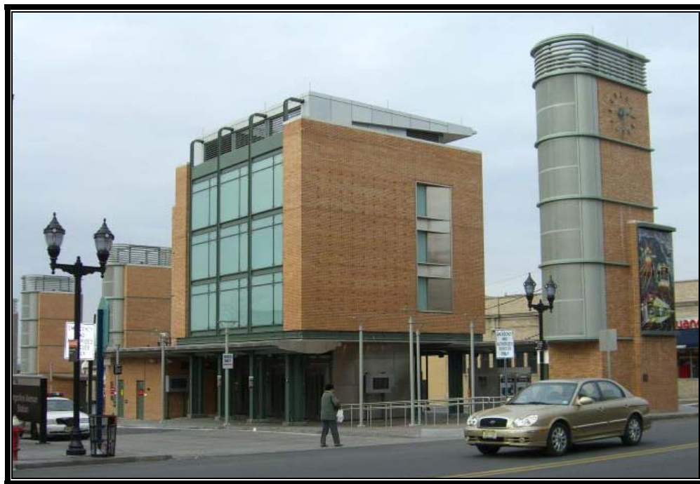
Bergenline Avenue Station in Union City surface entrance
