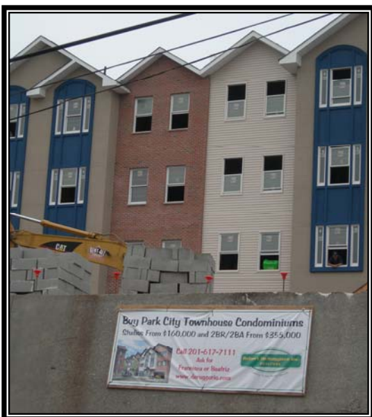
Park City Condominiums, Union City
